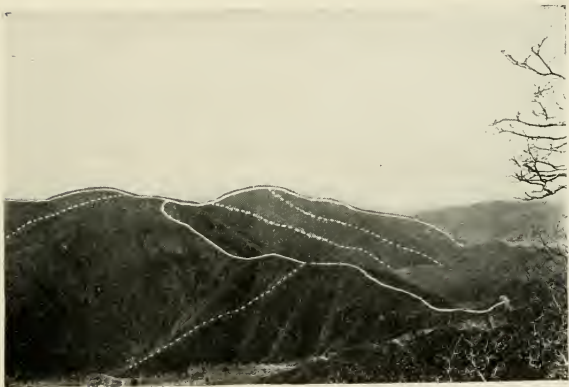
FIG. 60. - Location of Fire-Lines in the Angeles National Forest, California
